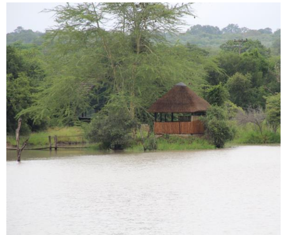
The bird hide on the Phelwana Dam has been re-thatched and re-roofed.
